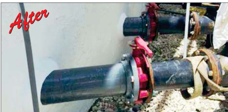
DuraQuartz LW used to repair the vertical tank wall.
