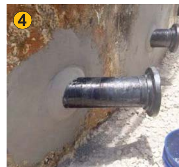
The repaired pipes and tank wall.
