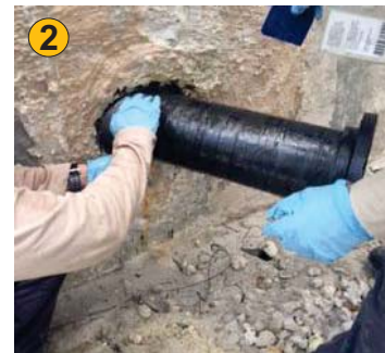
DuraWrap Carbon Fiber being applied.
