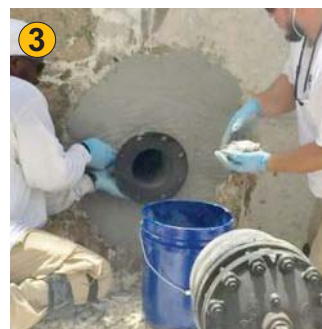
DuraQuartz LW used to repair the vertical tank wall.
