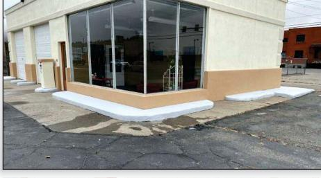
Damaged concrete curbs outside of a small Montana business were cracked and crumbling after years of expansion and contraction from freeze/thaw cycles. The local ENECON Distributor was called in to provide a solution.
