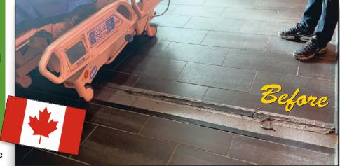
This floor expansion joint in one of the major hospitals in Montreal, Canada, needed to be replaced. Its condition was worsening every dav because of constant traffic in the hospital hallway. The hospital had to temporarily fix and then re-fix the joint almost every other day, with duct tape. This was creating a tripping hazard for patients and hospital staff.
